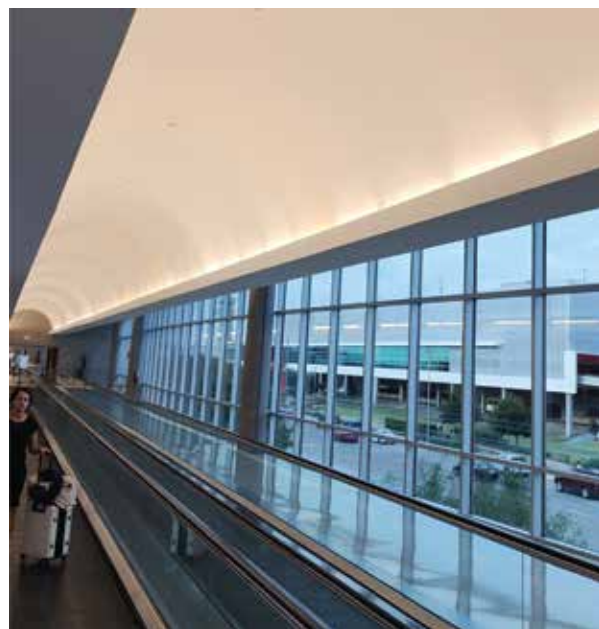
Fluorescent Bulbs create gaps in lighting
